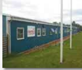
WR Controls Europe Timmele, Sweden
